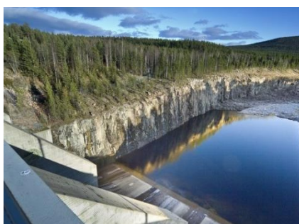
Power Generation -Generation
