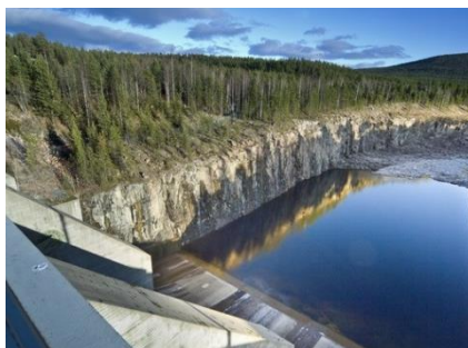
Power Generation -Generation
