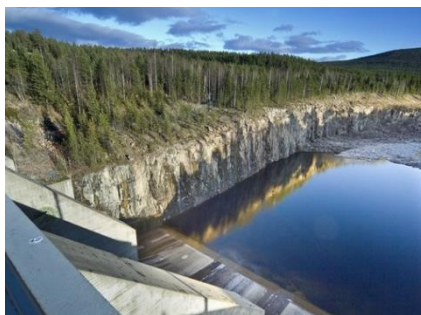
Power Generation -Generation
