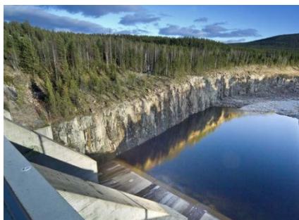
Power Generation -Generation
