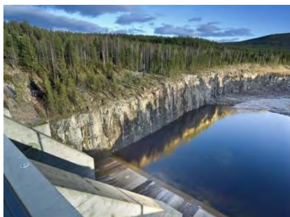
Power Generation -Generation
